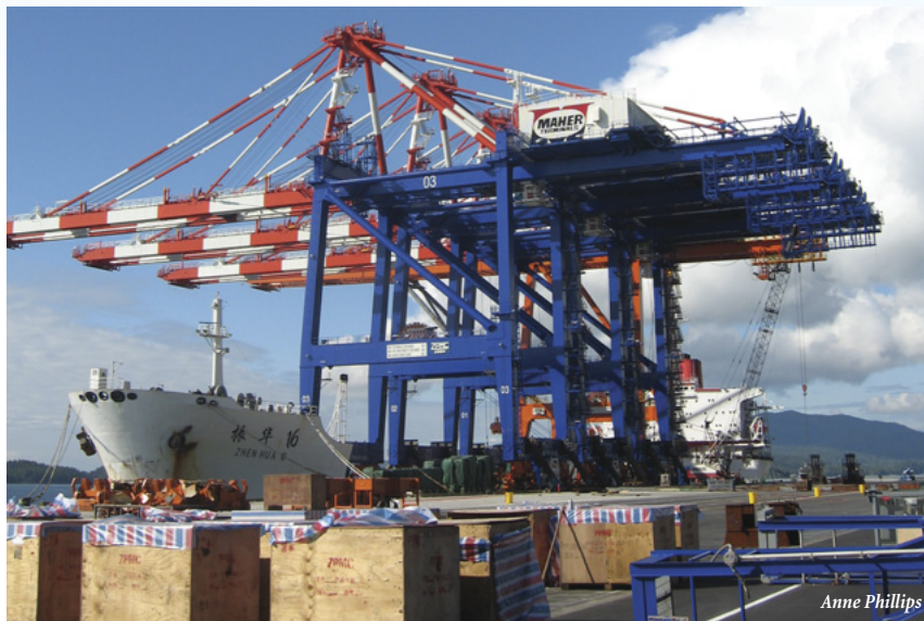
Container cranes shipped from China, await offloading and positioning to function at the new Fairview Container Terminal at the Port of Prince Rupert, BC.
