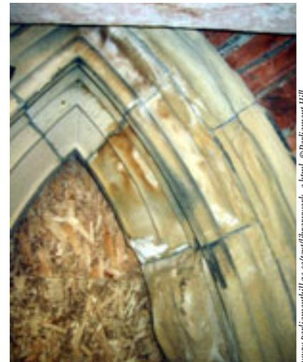
Example of damage (efflorescence – seen as a powdery deposit) on the stone arches.
